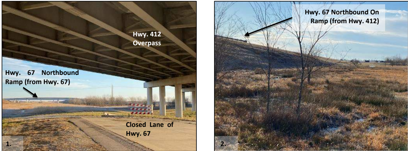
Figure 33: Existing Hwy. 67 at the Hwy. 67/Hwy. 412 Interchange at Start of Alternatives 2 and 3
