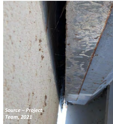
Figure 24: Bridge Joint at Hwy. 412
