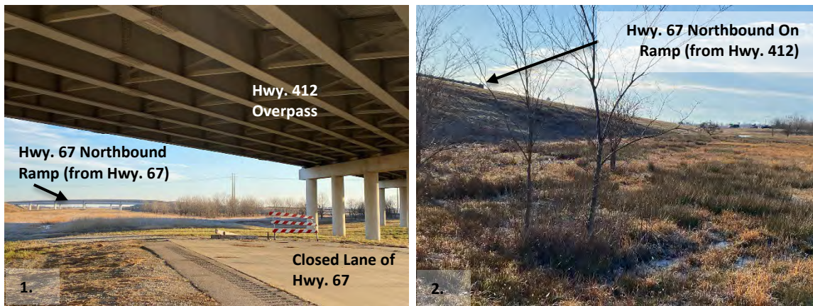
Figure 3: Existing Hwy. 67 at the Hwy. 67/Hwy. 412 Interchange at Start of Alternatives 2 and 3
