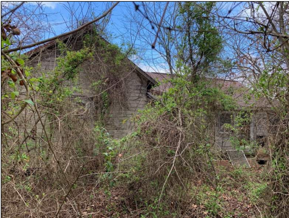
Figure 9. Property 21 view west (IMG_2536).
