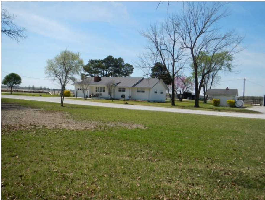
Figure 2-13. Property 1 front façade, well house, view southwest (DSCN1599).
