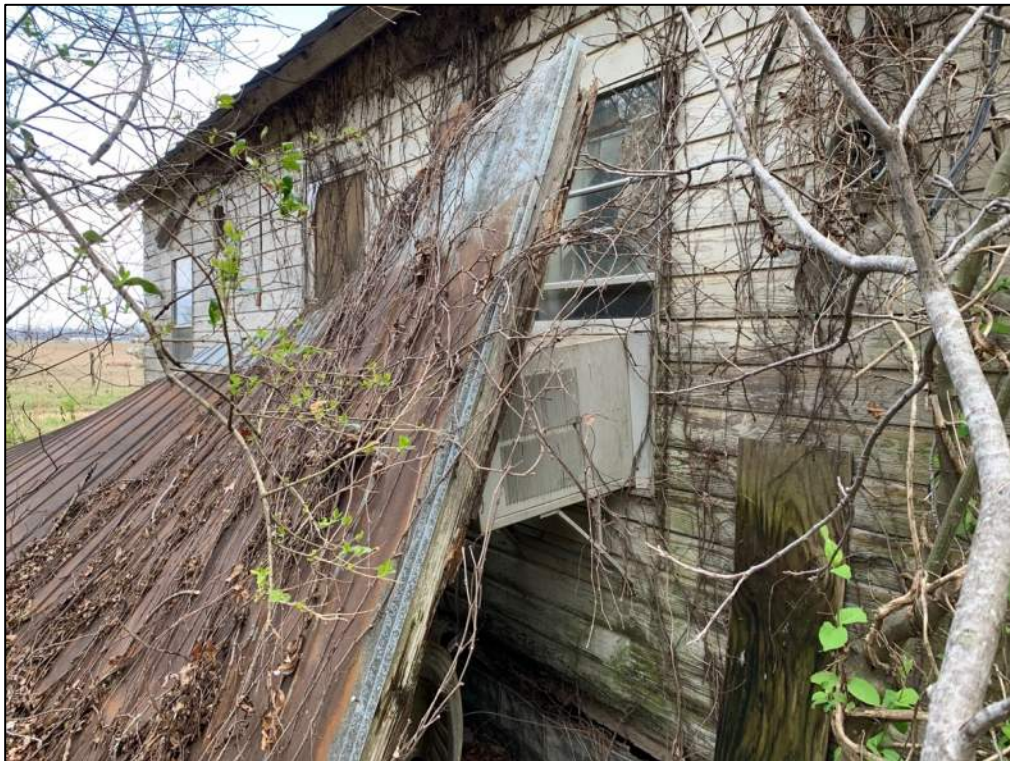
Figure 11. Property 21 view west (IMG_2539).
