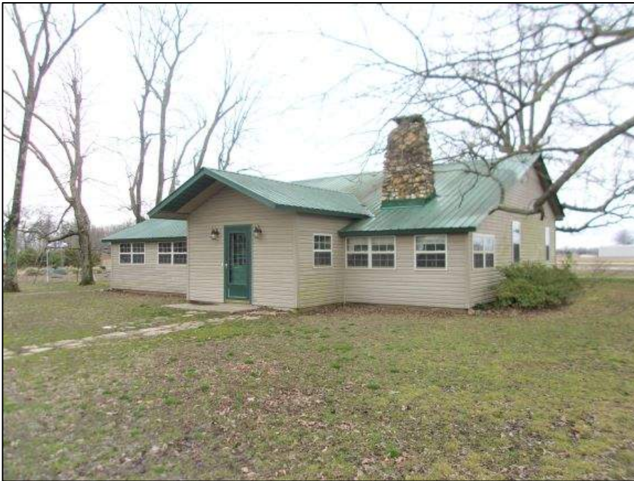
Figure 2-86. Property 20a, main house, view southwest (assessors office photo).
