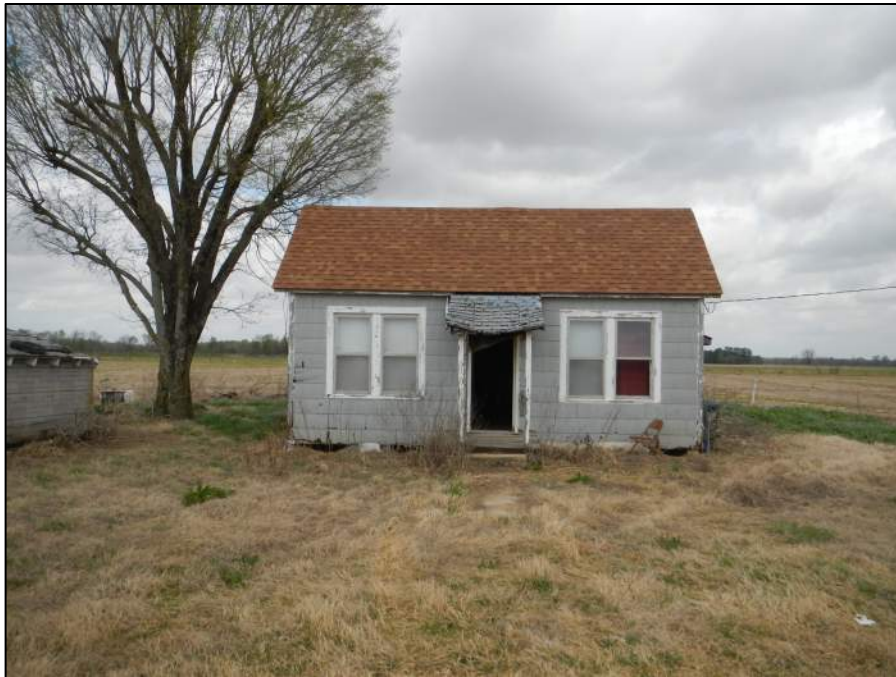
Figure 2-53. Property 11, front façade, view north (DSCN1645).
