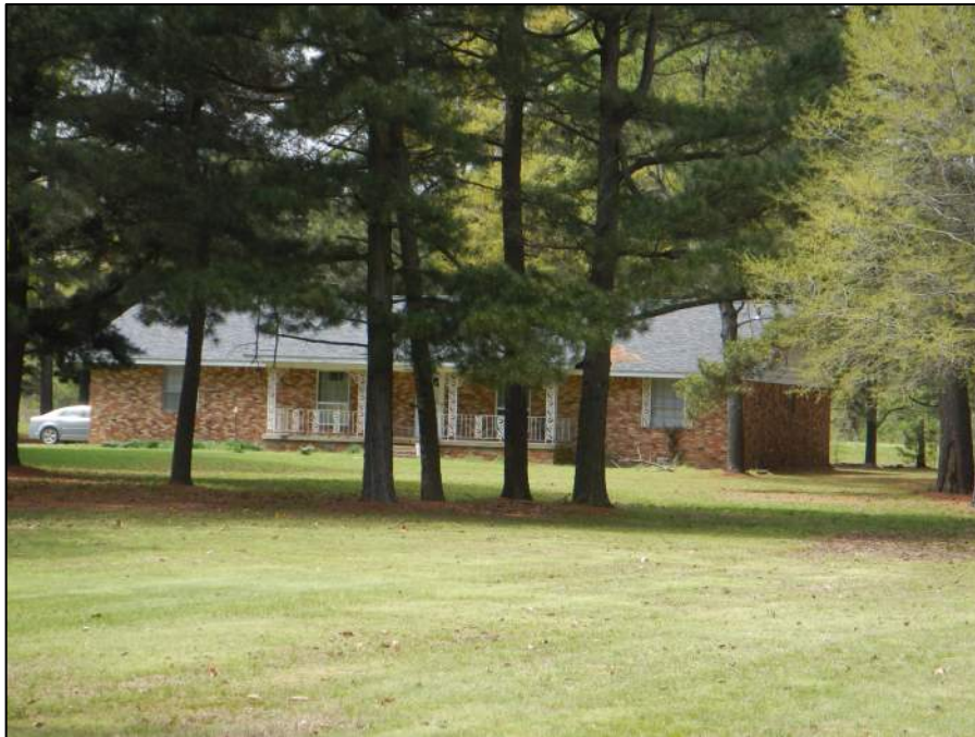
Figure 2-65. Property 13, view west, close-up 2 (DSCN1660).
