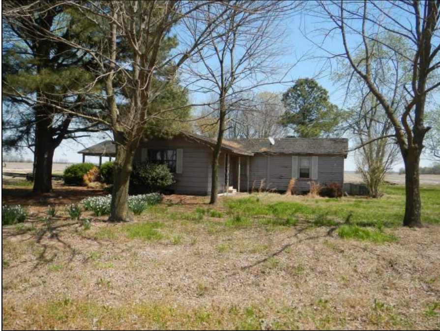
Figure 2-25. Property 3, front façade and yard, view east-northeast (DSCN1592).
