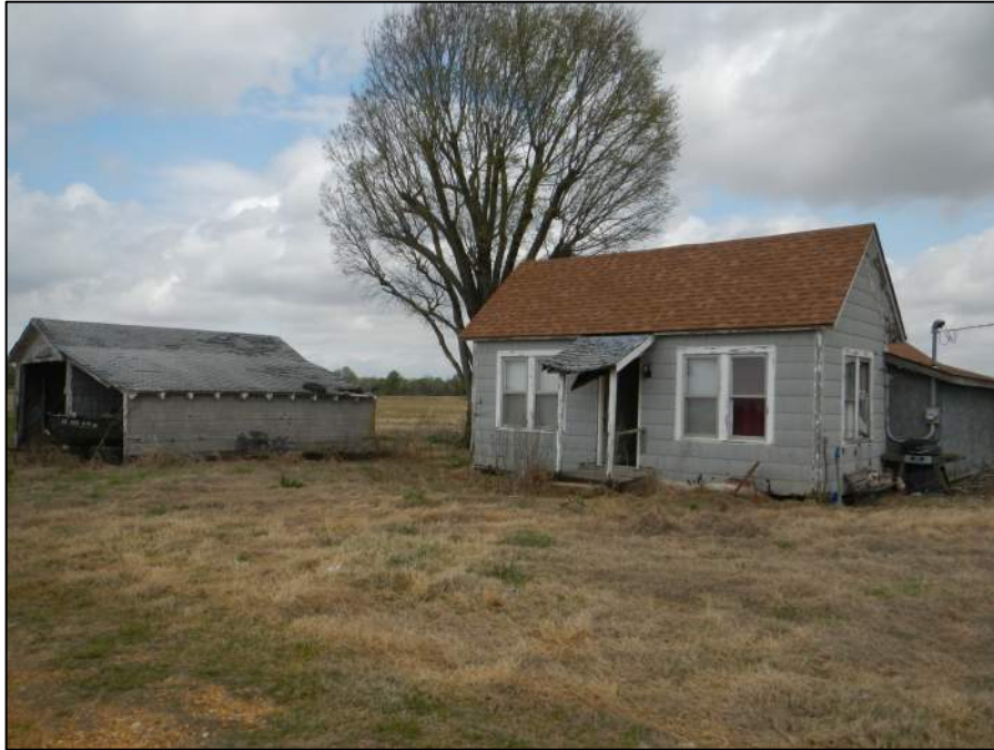
Figure 2-52. Property 11, house and garage, view northwest (DSCN1644).
