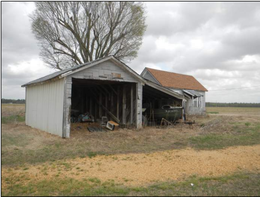
Figure 2-55. Property 11, garage, view northeast (DSCN1647).
