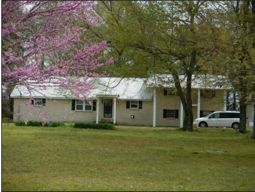
Figure 2-66. Property 14, view east (DCNS1661).
