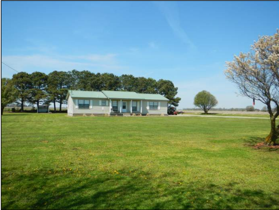
Figure 2-37. Property 6, view northwest (DSCN1580).
