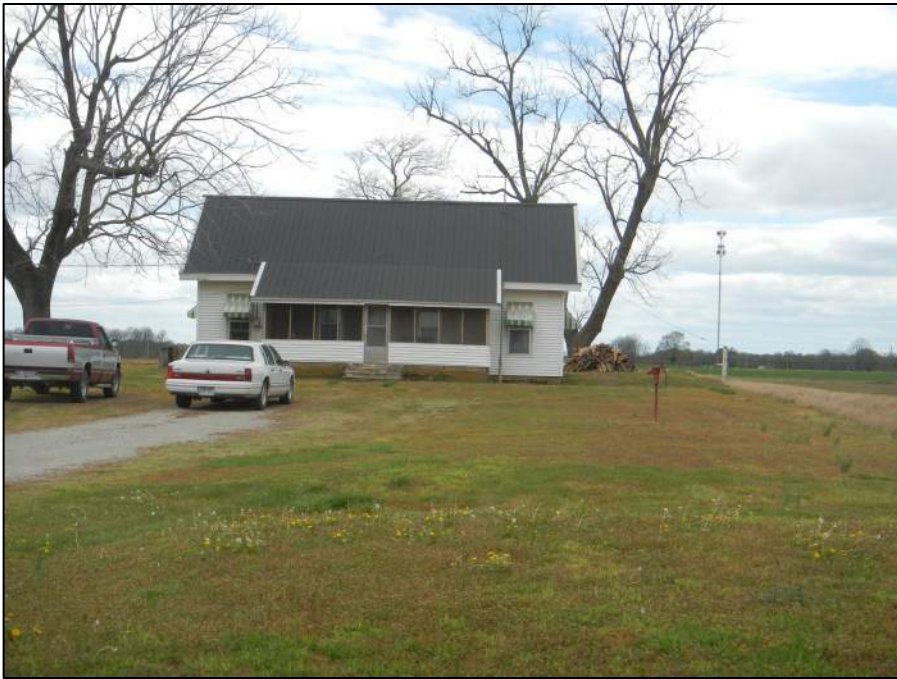
Figure 2-174. Property 35 house, view west (DSCN1747).
