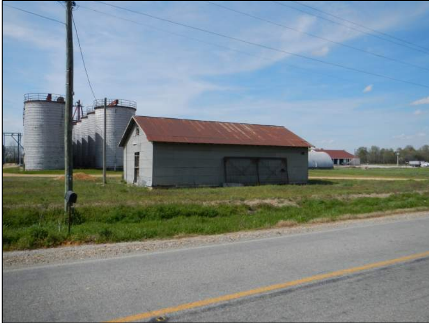
Figure 1-16. NRHP-eligible Knobel Grain facility (CY0079) in Knobel, view northwest (DSCN 1622).
