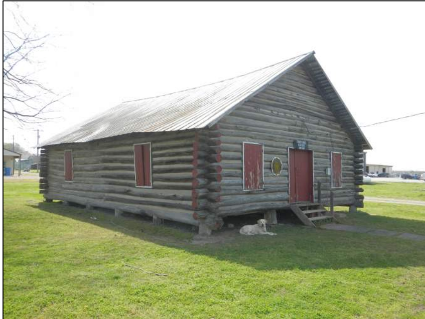
Figure 1-10. NRHP-listed American Legion Post No. 72 (CY0071) in Knobel, view west (DSCN 1627).
