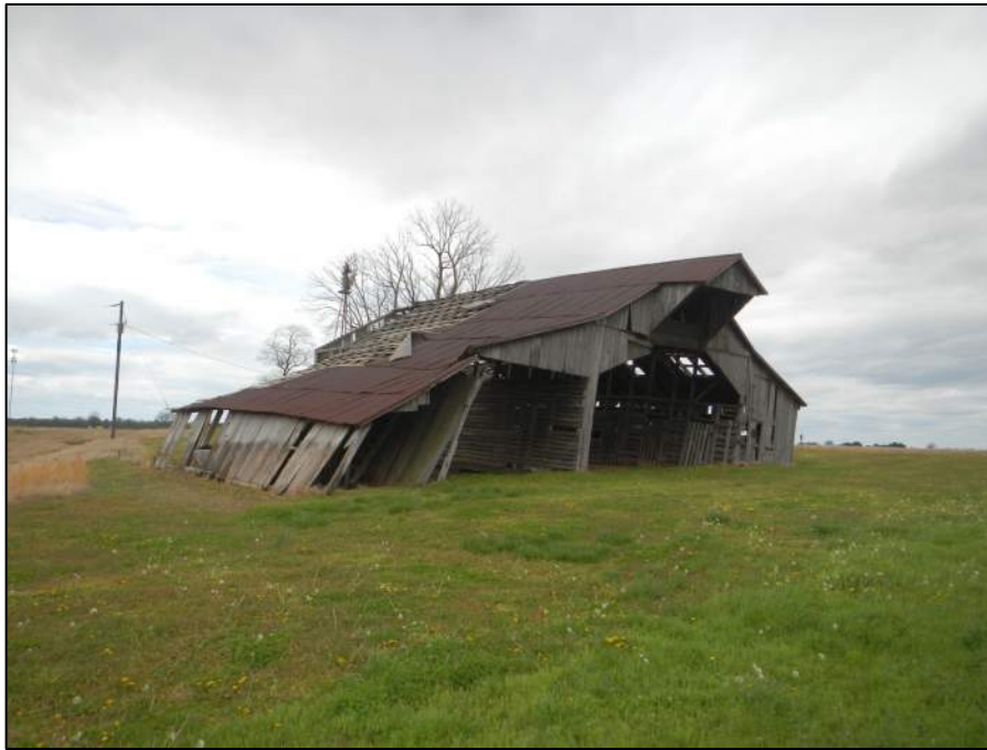
Figure 2-170. Property 35 barn, view northwest (DSCN1743).
