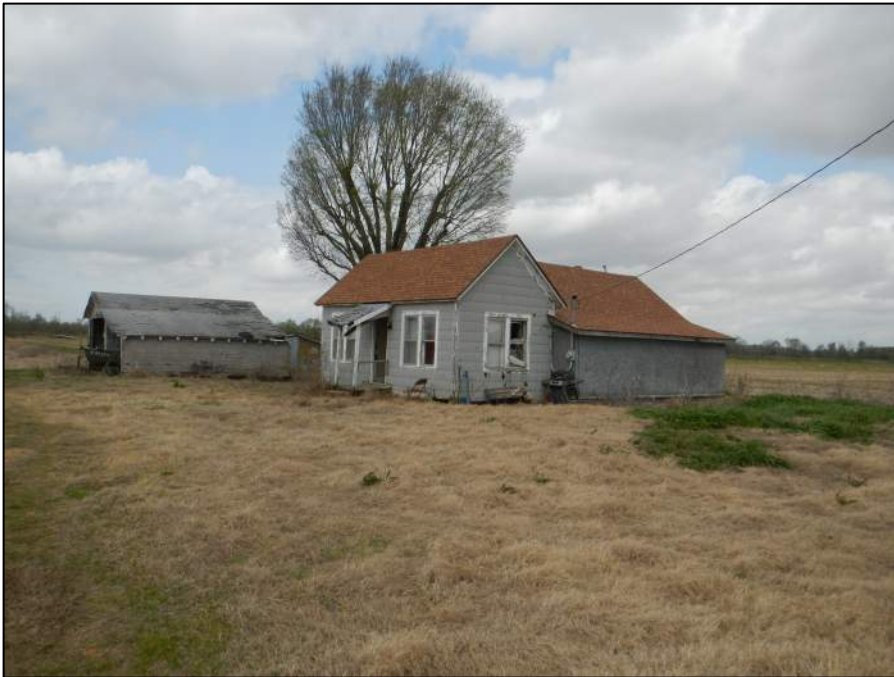
Figure 2-51. Property 11, view northwest (DSCN1643).
