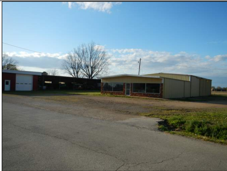
Figure 1-17. NRHP-ineligible MOARK Depot (CY0080) north of Corning, view northwest (DSCN 1796).
