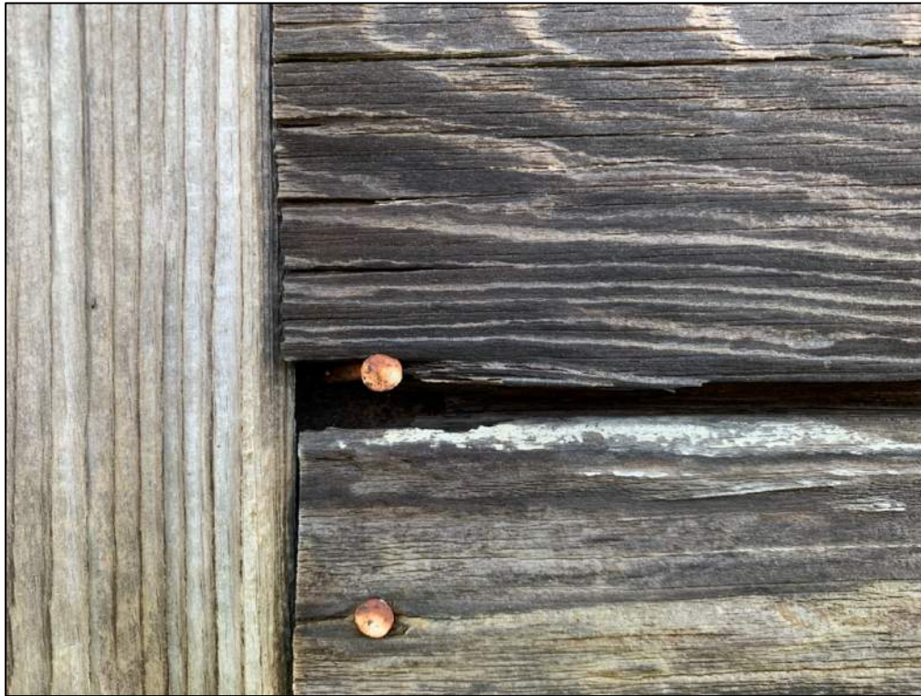
Figure 14. Property 21 exterior detail showing wire nails (IMG_2552).
