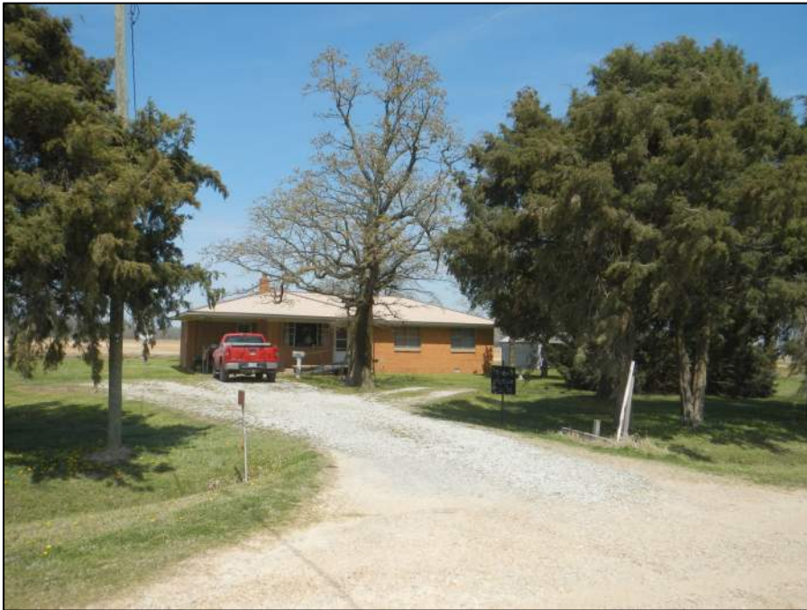
Figure 2-30. Property 4, front façade, view north (DSCN1606).
