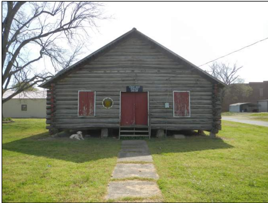
Figure 1-09. NRHP-listed American Legion Post No. 72 (CY0071) in Knobel, front façade, view southwest (DSCN 1625).
