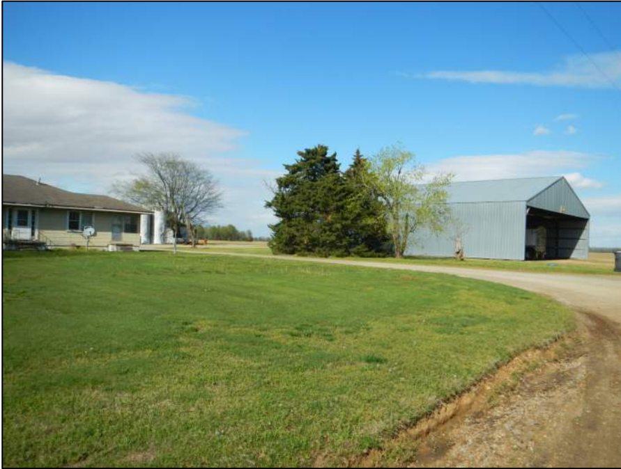
Figure 2-182. Property 37, view northeast (DSCN1777).
