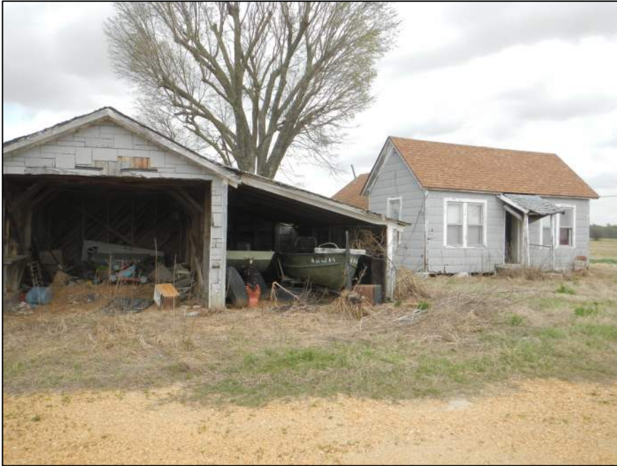
Figure 2-54. Property 11, garage and main house, view northeast (DSCN1646).
