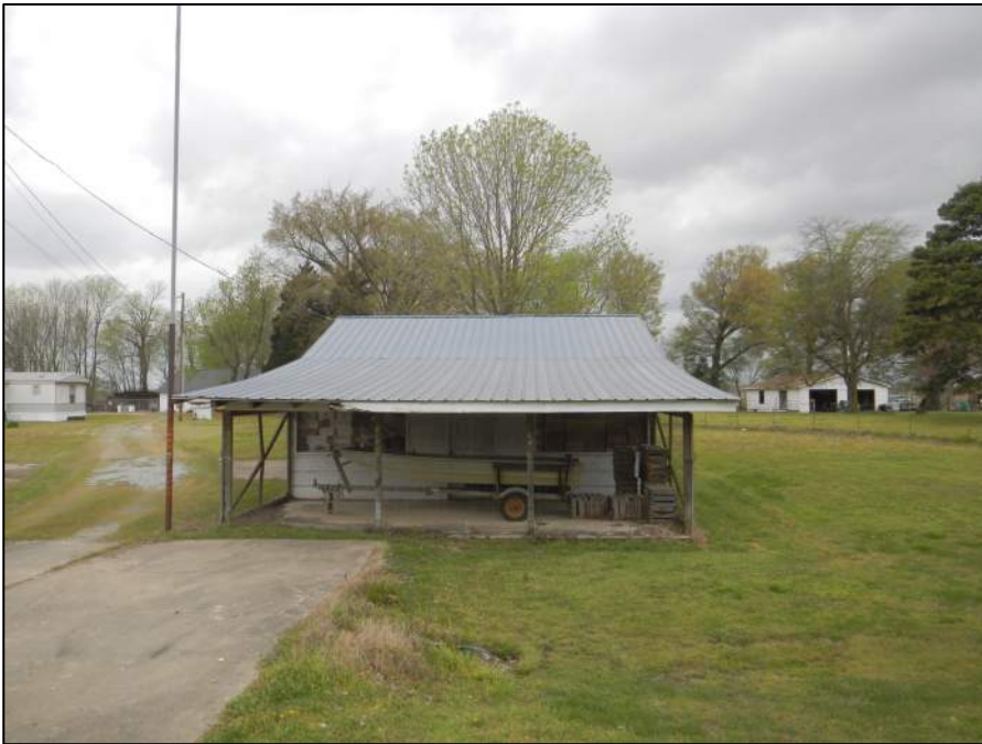
Figure 2-147. Properties 30-3 and 2 (rear), view west (DSCN1702).
