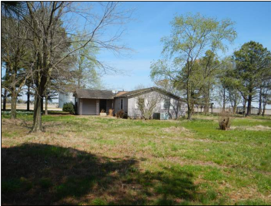
Figure 2-26. Property 3, south façade and yard, view north (DSCN1594).
