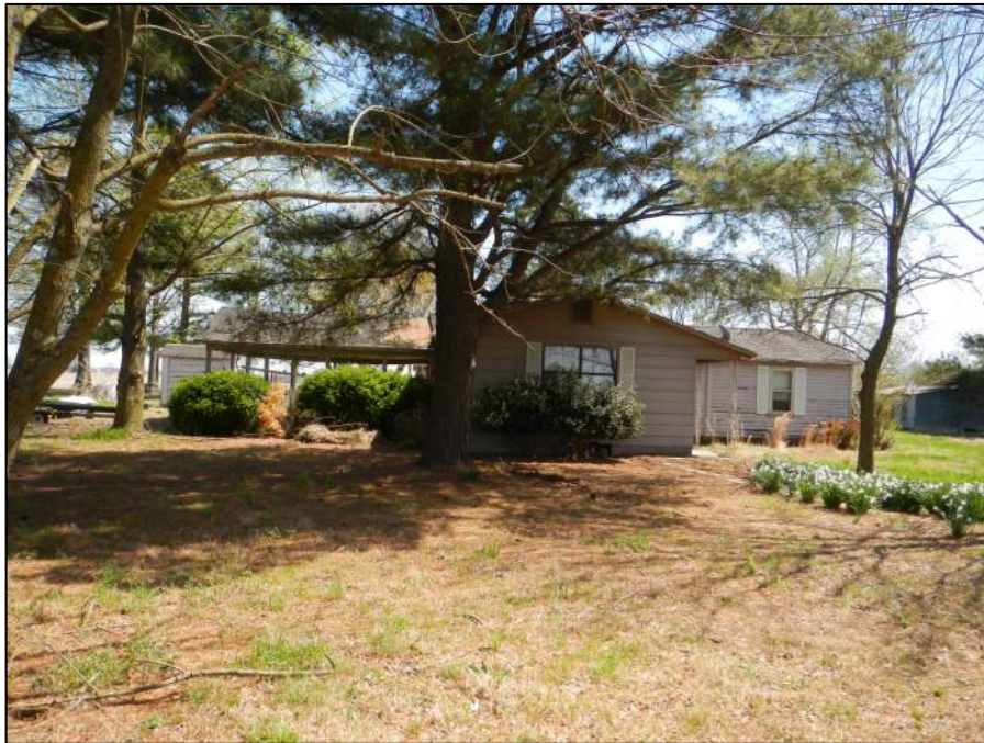
Figure 2-24. Property 3, front façade and yard, view east (DSCN1591).
