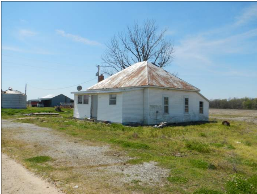
Figure 2-19. Property 2, oblique view southwest (DSCN1585).
