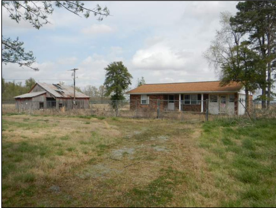
Figure 2-118. Property 27, view northeast (DSCN1687).
