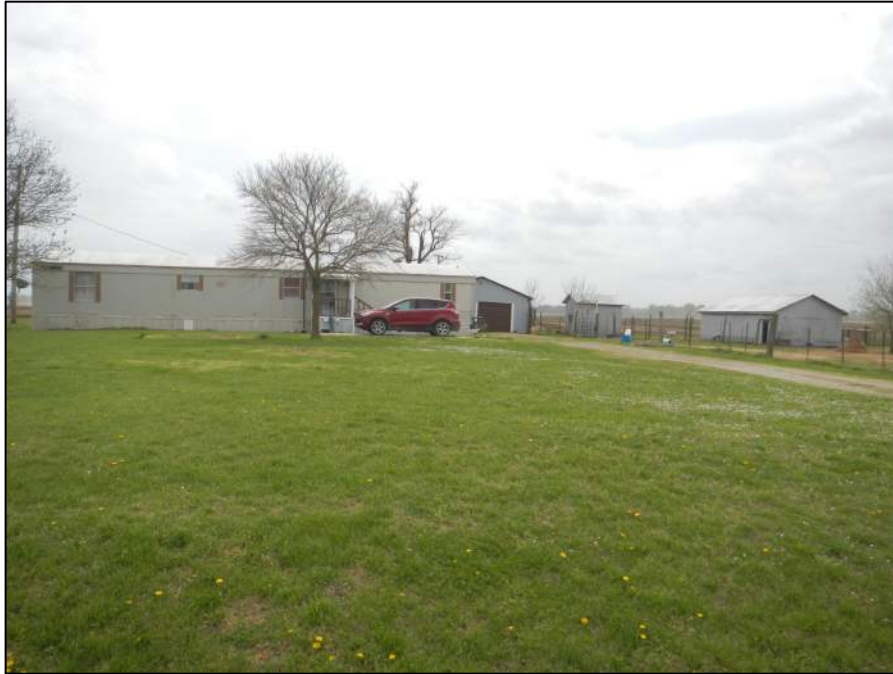
Figure 2-96. Trailer east of Property 22, view south (DSCN1666).
