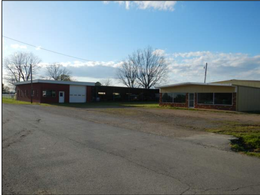
Figure 1-18. NRHP-ineligible MOARK Depot (CY0080) north of Corning, view northwest (DSCN 1797).
