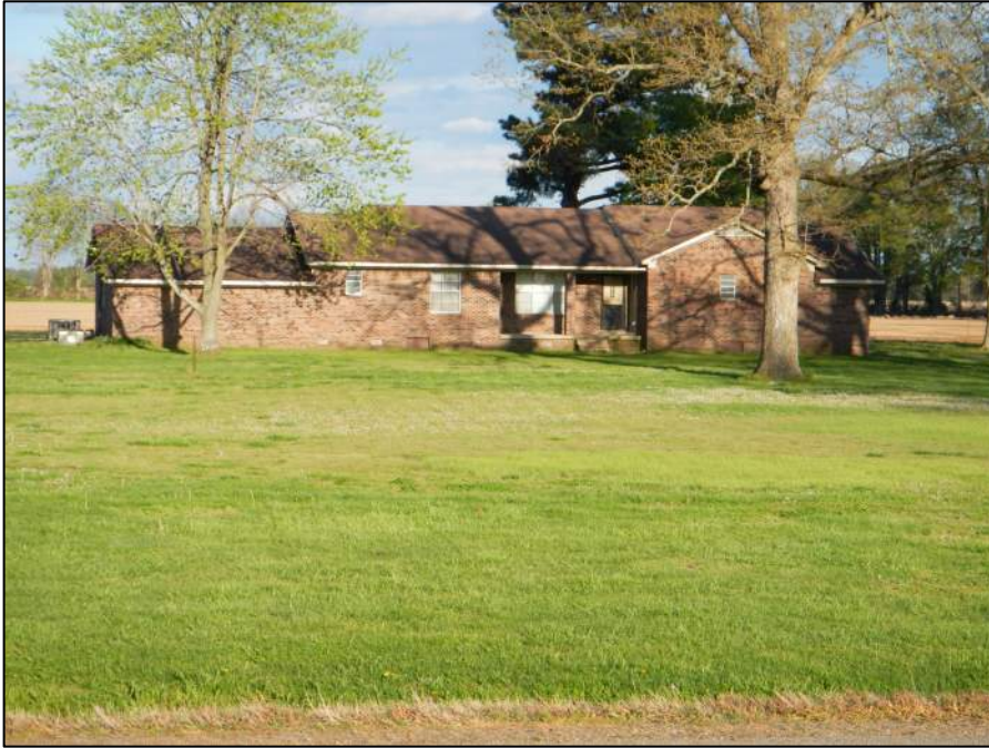
Figure 2-72. Property 16, view east (DCNS1808).
