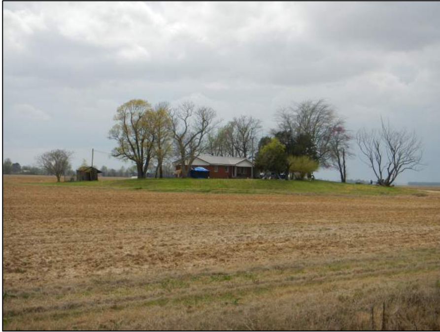
Figure 2-135. Property 29b, view southwest (DSCN1683).
