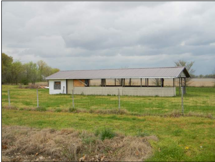
Figure 2-138. Property 30-1, view west (DSCN1690).
