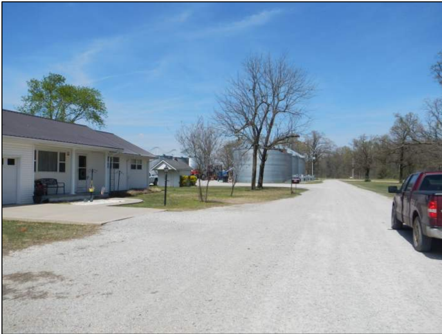
Figure 2-17. Property 1 main house, grain silos, view north (DSCN1603).
