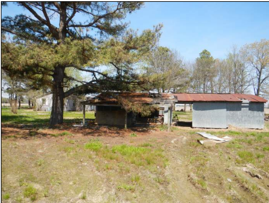
Figure 2-28. Property 3, barn/shed and main house, view north (DSCN1597).
