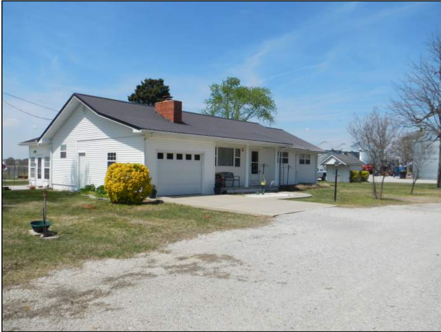
Figure 2-16. Property 1 main house, well spigot, grain silos, view northwest (DSCN1603).
