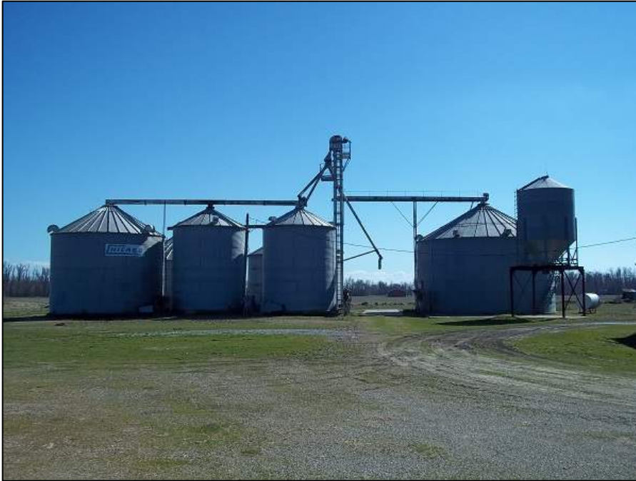
Figure 2-80. Property 18, grain silos, view south (assessors office photo).
