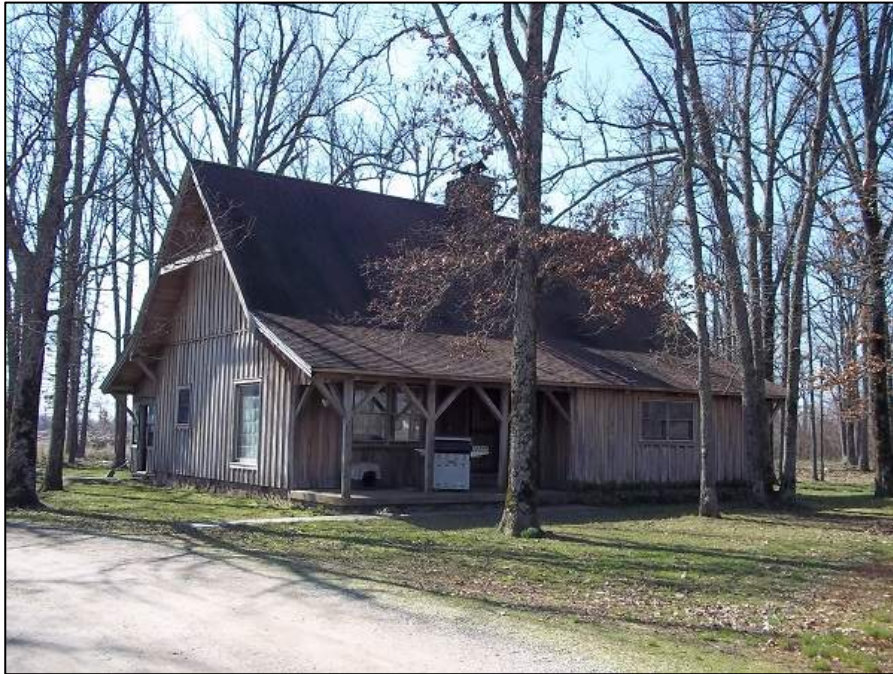
Figure 2-87. Property 20b, main house, view southwest (assessors office photo).
