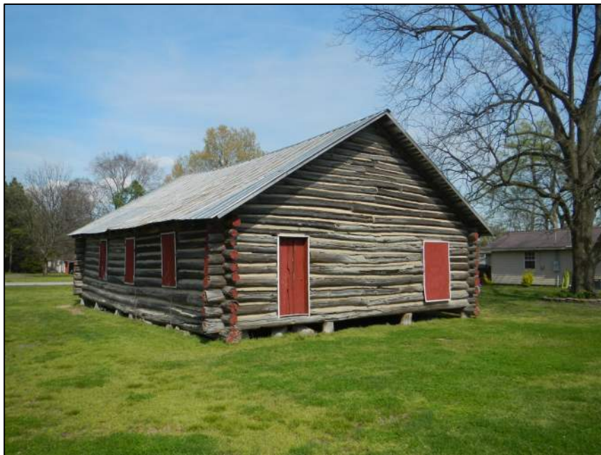
Figure 1-11. NRHP-listed American Legion Post No. 72 (CY0071) in Knobel, view northeast (DSCN 1628).
