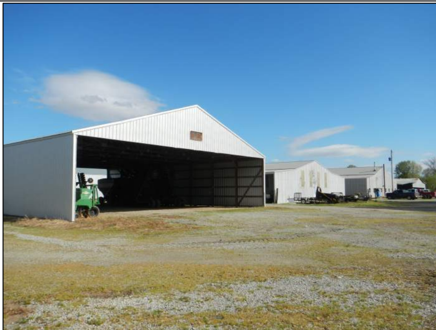
Figure 2-177. Property 37, view south-southeast (DSCN1772).
