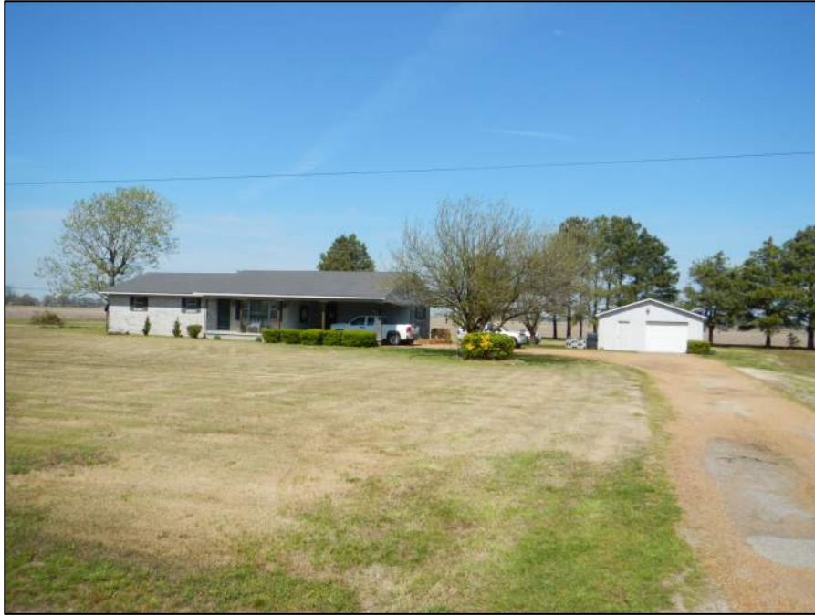
Figure 2-150. Property 31, view west (DSCN1561).
