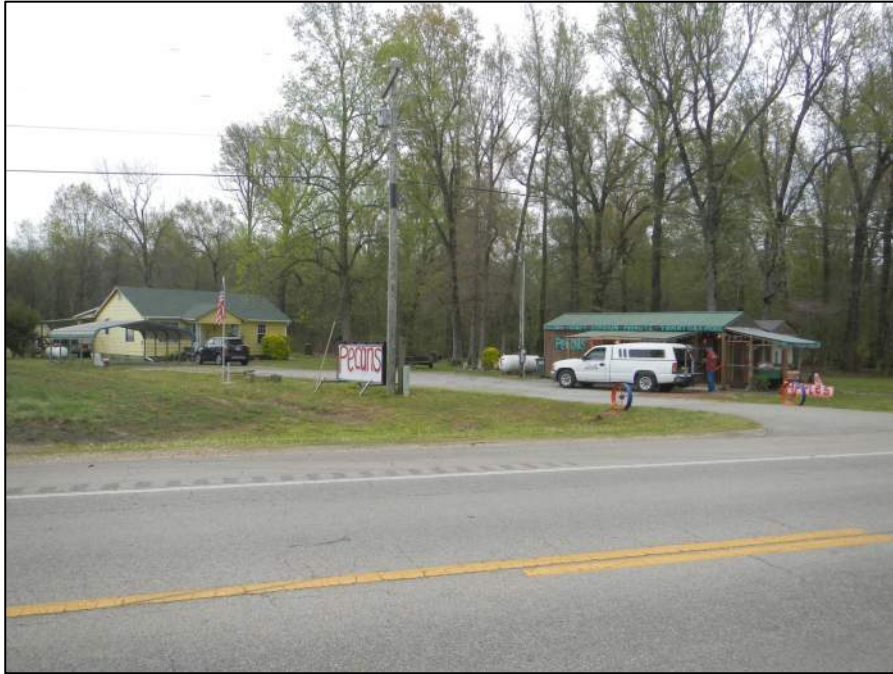
Figure 2-124. Property 29a-1, view east (DSCN1692).
