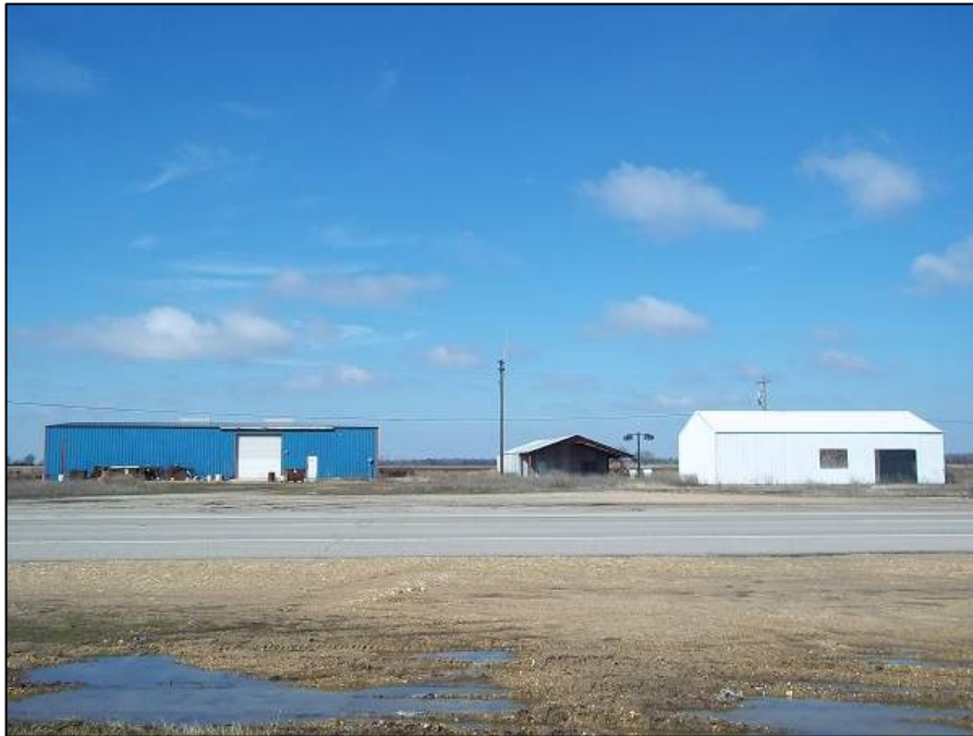
Figure 2-115. Property 26, view west of southern buildings (assessors office photo).
