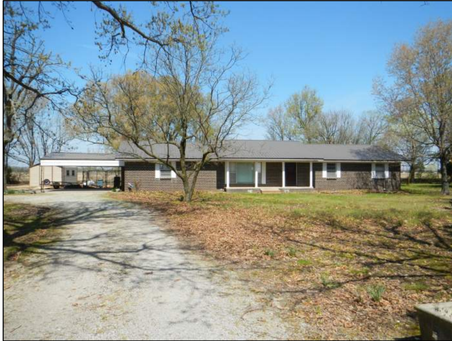
Figure 2-154. Property 32, view west (DSCN1562).
