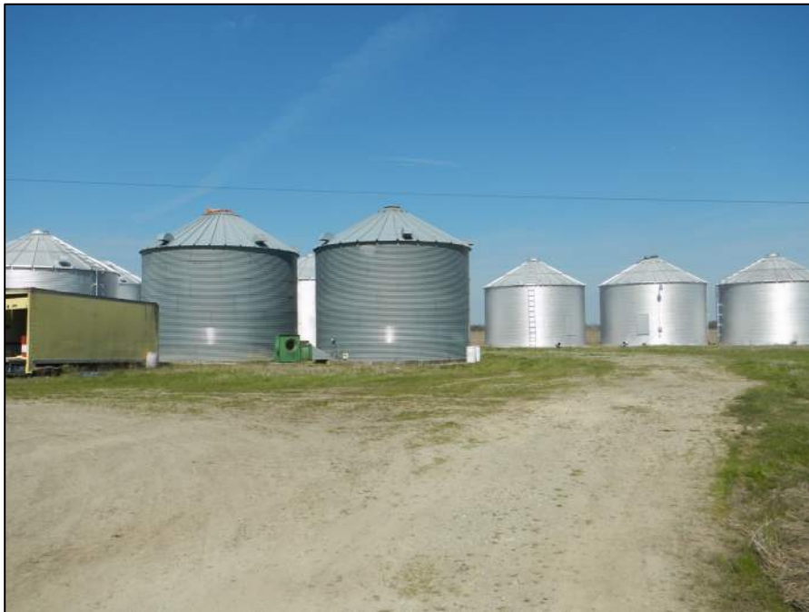
Figure 2-153. Property 31, view northwest of silos (DSCN1559).
