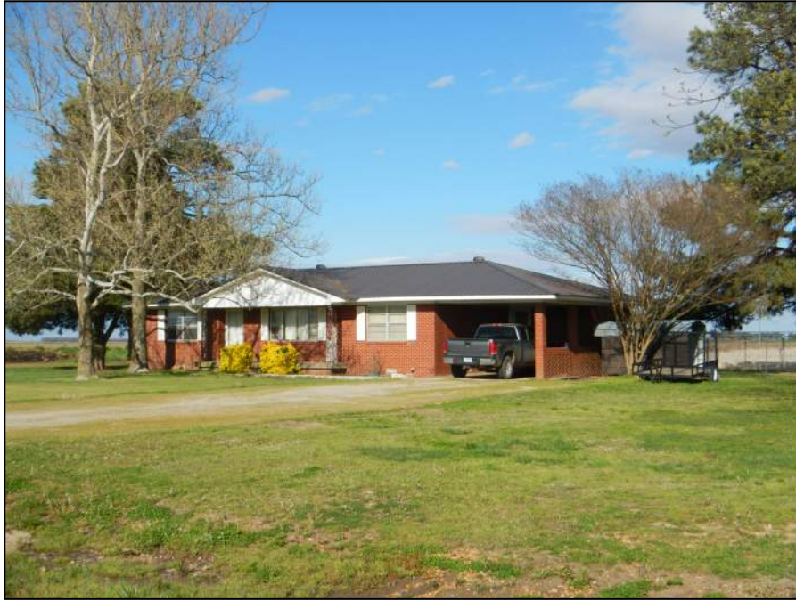
Figure 2-184. Property 38, view northeast (DSCN1783).
