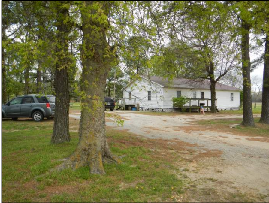
Figure 2-60. Property 12, oblique view northeast (DSCN1655).
