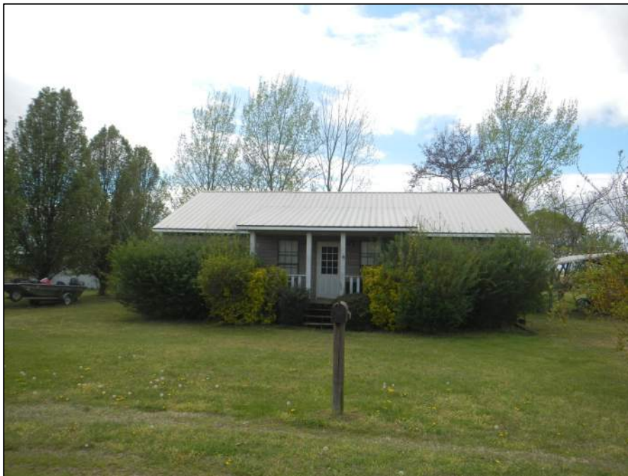
Figure 2-176. Property 36, view west (DSCN1749).
