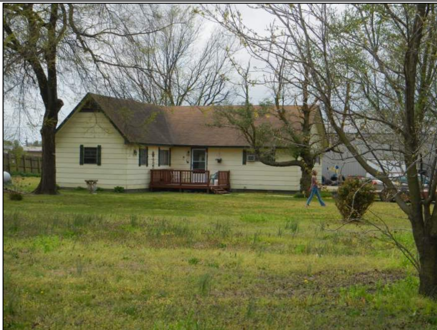
Figure 2-101. Property 24, view west (DSCN1672).
